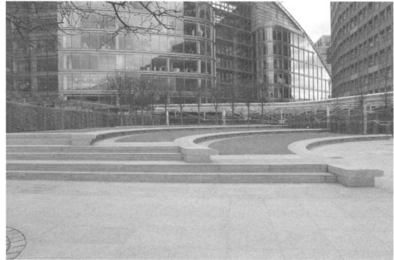
Plate 1 Green roof garden in Cardinal Place, Victoria; part of the Victoria BID green infrastructure expansion project Source: Sarah Jones, 14 April 2013
